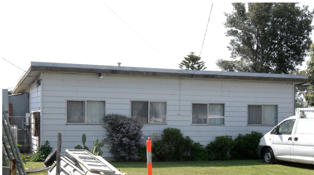
Figure 4. The front façade of 108 George Street (Source: Context, 2017)
