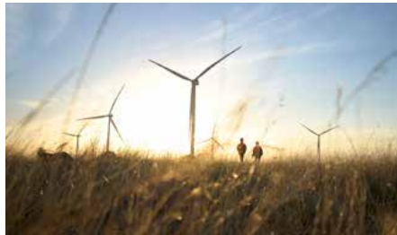
Dundonnell Wind Farm image courtesy of Tilt Renewables Australia Pty Ltd
